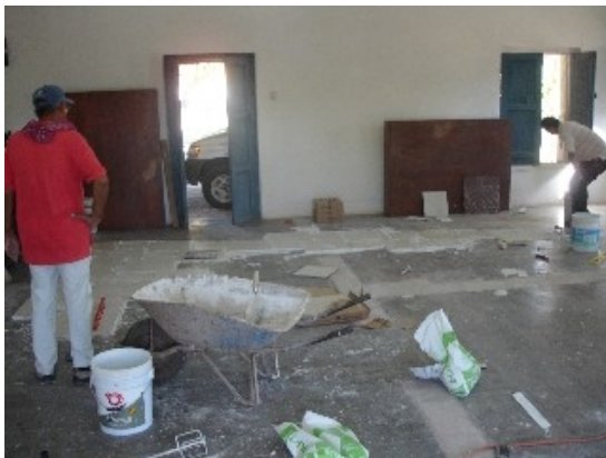
End of November - main room
